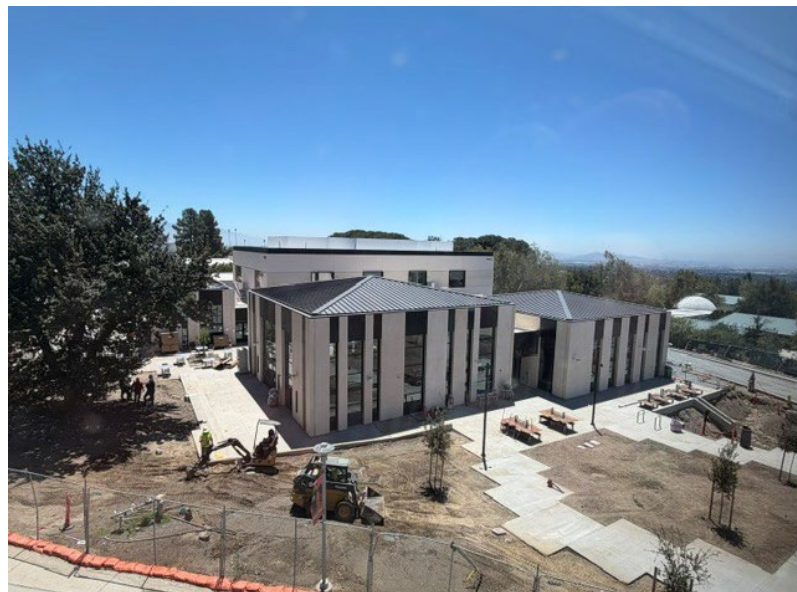
RANCHO CUCAMONGA MACC RENOVATION & ADDITION In Construction
