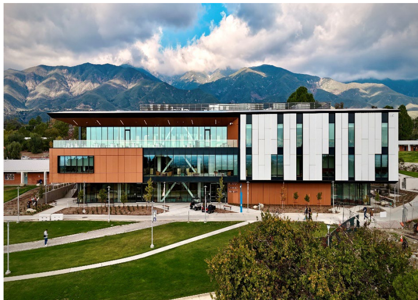
RANCHO CUCAMONGA LLC (LIBRARY LEARNING COMMONS) Completed
