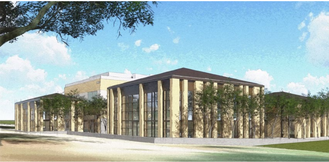
RANCHO MACC Renovation & Addition
