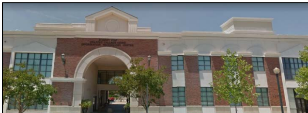
ROBERT PILE INFORMATION TECHNOLOGY CENTER 13170 Seventh Street, Chino
