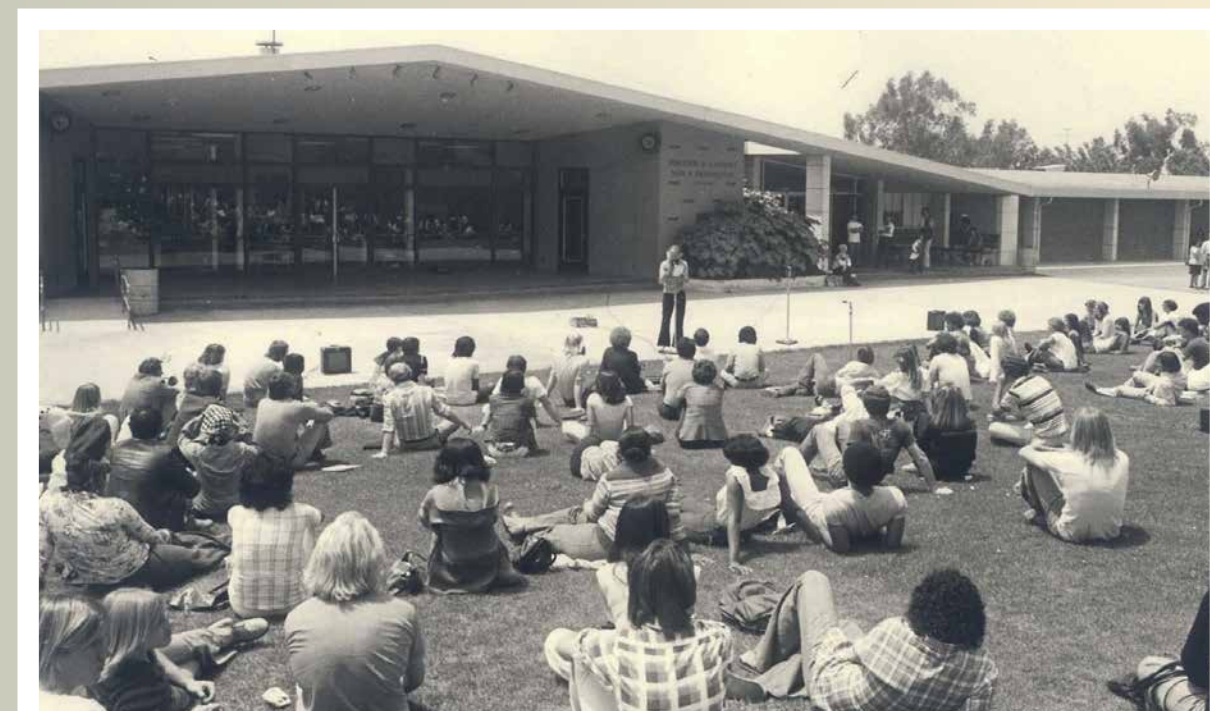
DOMESTIC SCALE: Most of the original buildings were single story with a low gable roof, typical of suburban residential architecture of the era. Here, students gather at the Campus Center.
