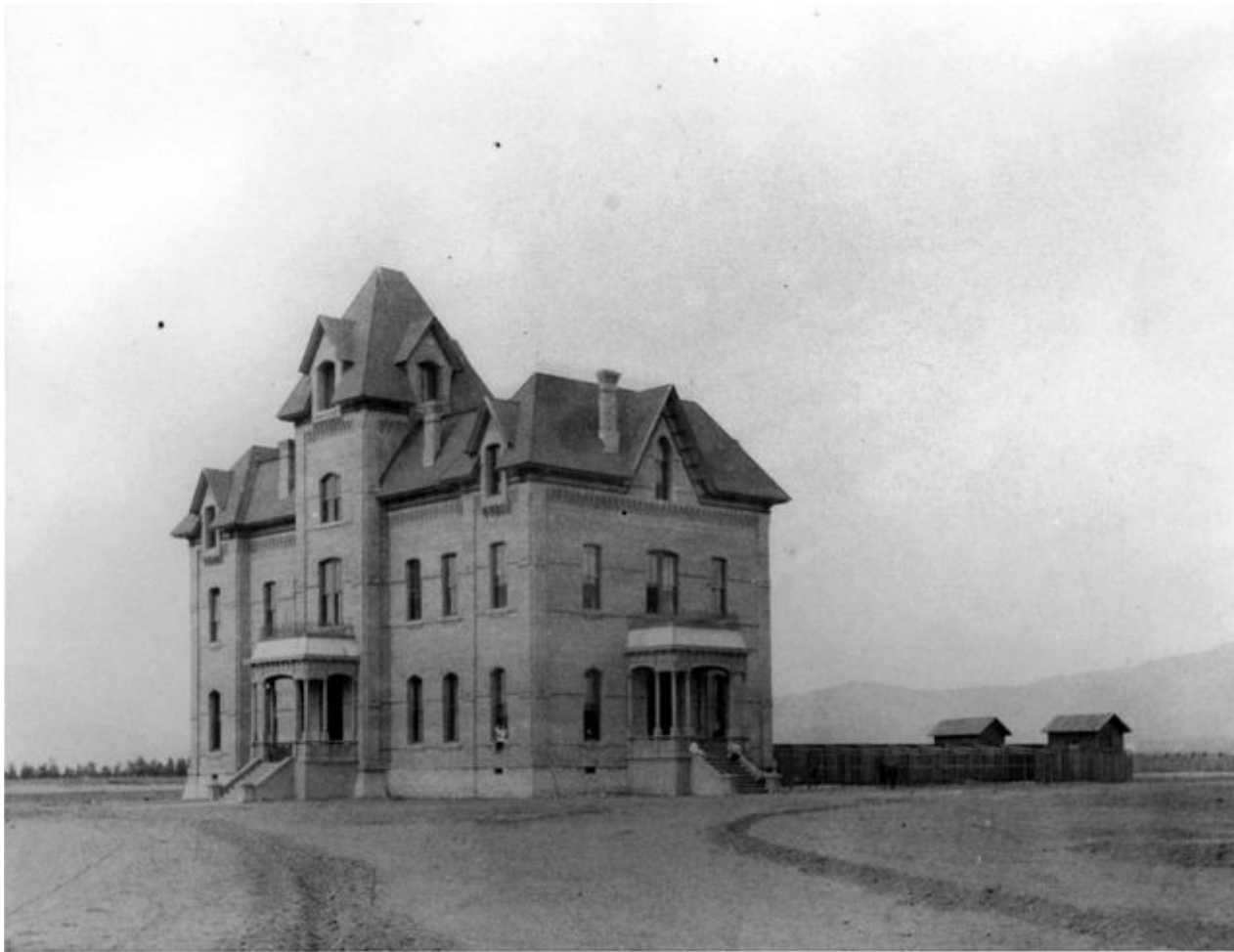
HMC ARCHITECTS + WHITEHALL PLACE
