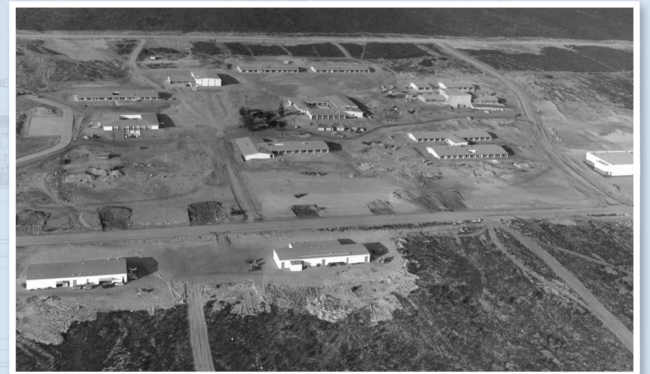
IN PROGRESS: Chaffey College under construction, ca. 1959, with all major buildings completed.
