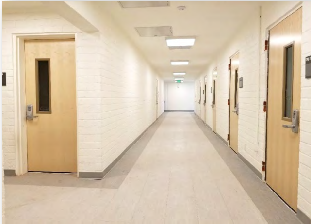
Theatre Wings Renovation - East and West Project Budget : $ 4,298,107
