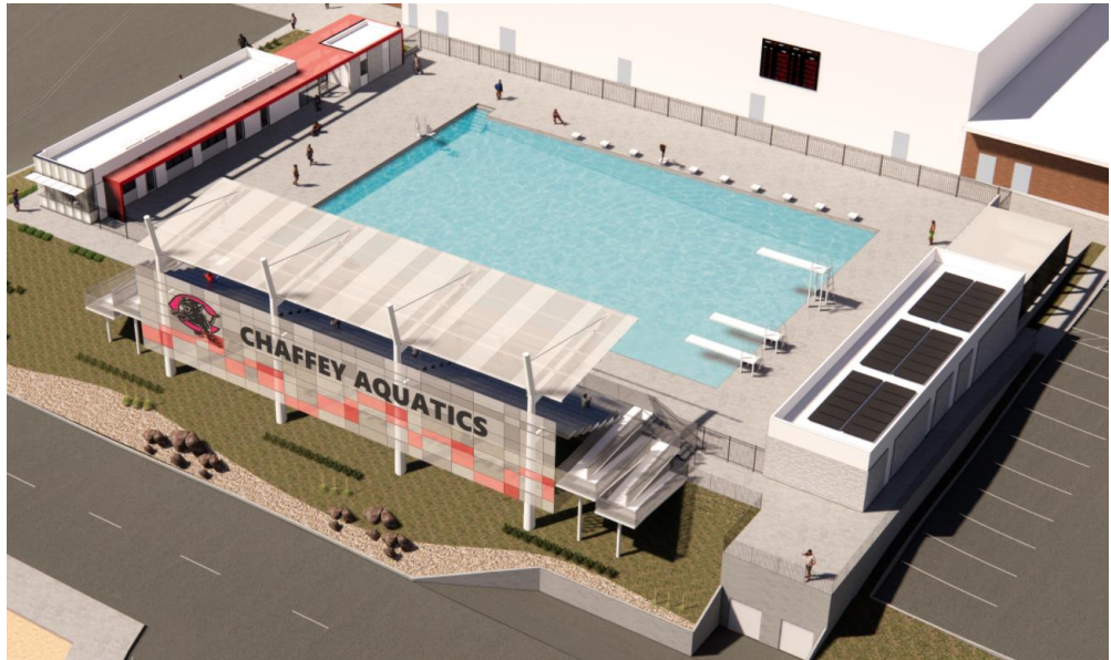
RANCHO CUCAMONGA Pool Renovation
