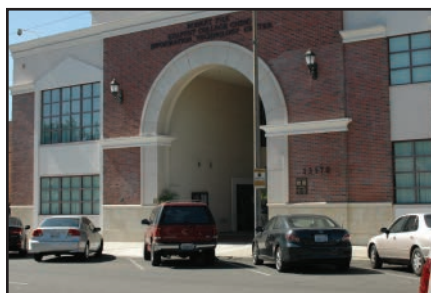
ROBERT PILE INFORMATION TECHNOLOGY CENTER 13170 Seventh Street, Chino
