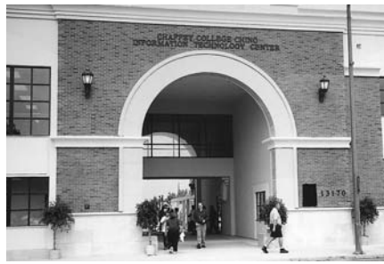
ROBERT PILE INFORMATION TECHNOLOGY CENTER 13170 Seventh Street, Chino
