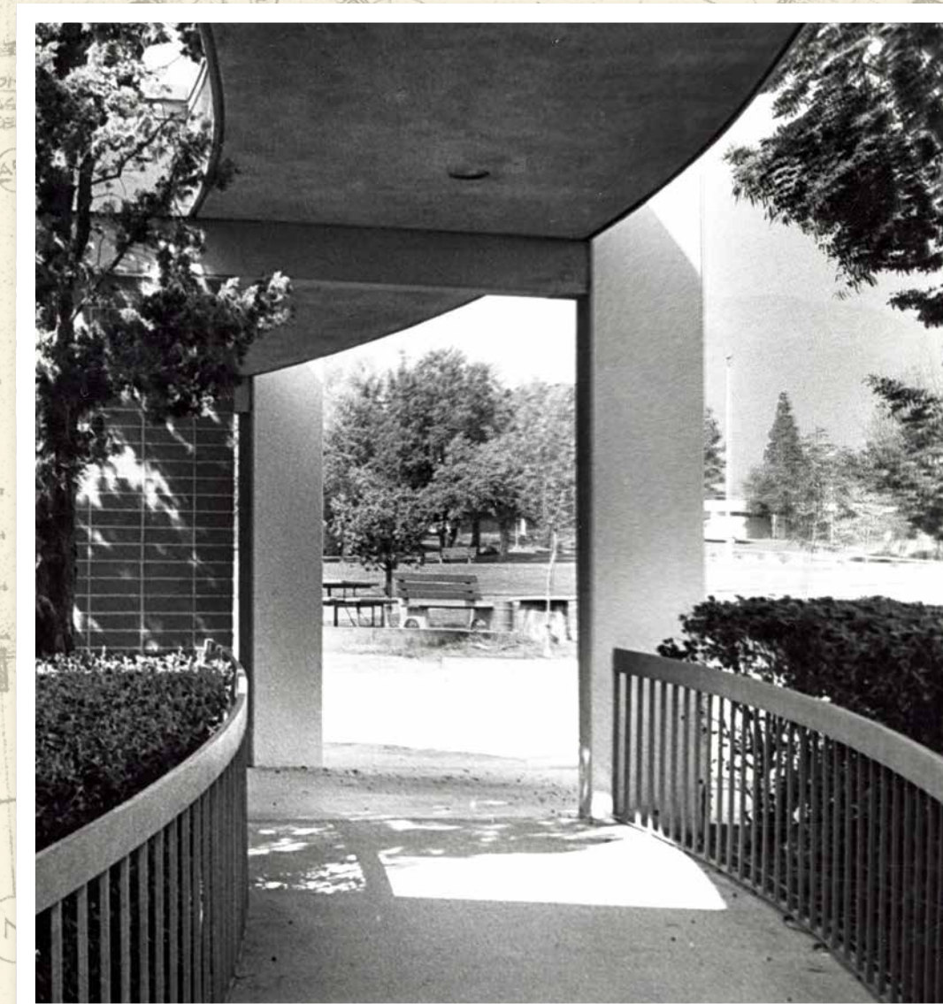
Open corridor formed by concrete piers and flat roof.
