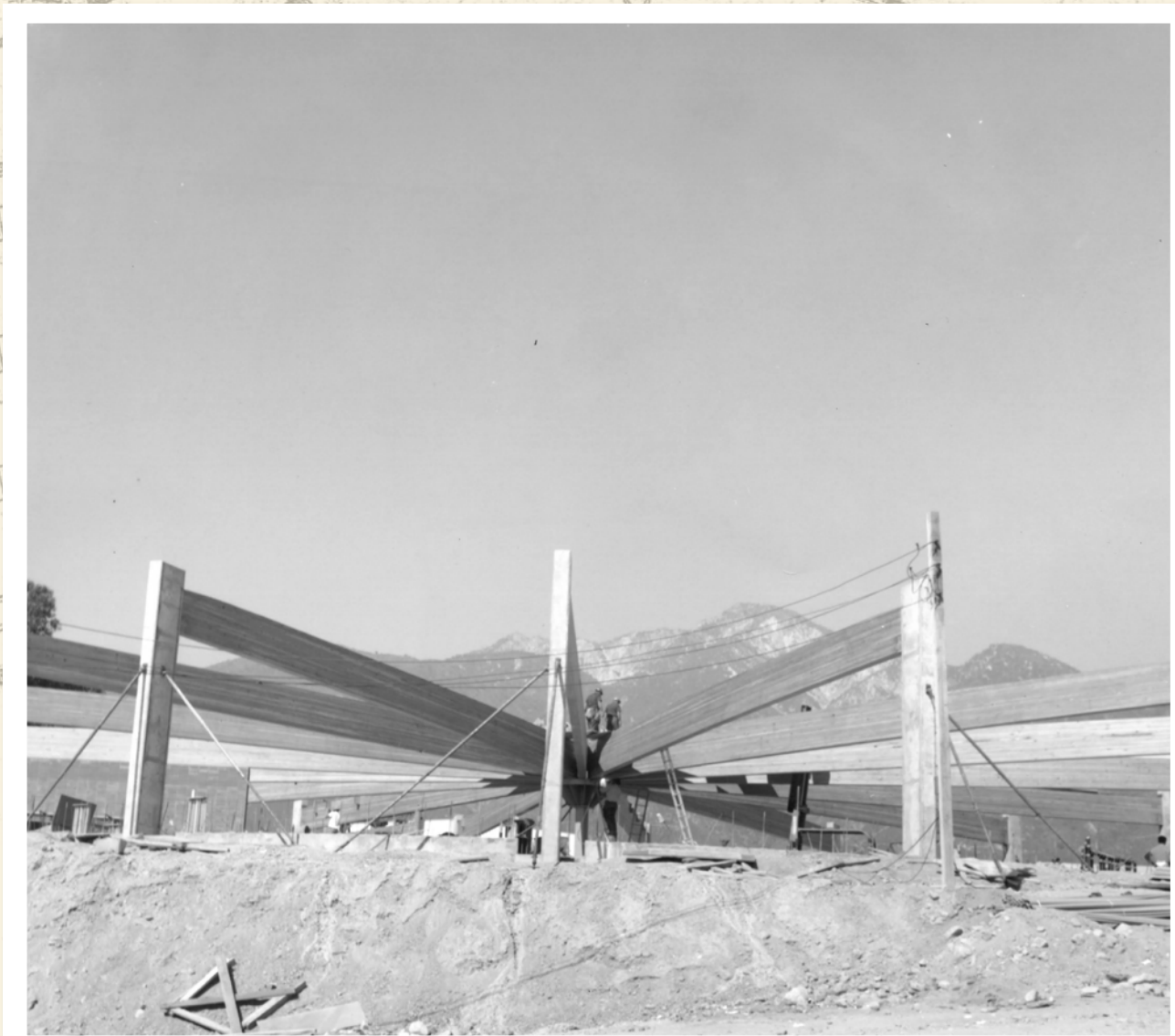
Laminated wood beams connect the concrete piers to a central hub.
