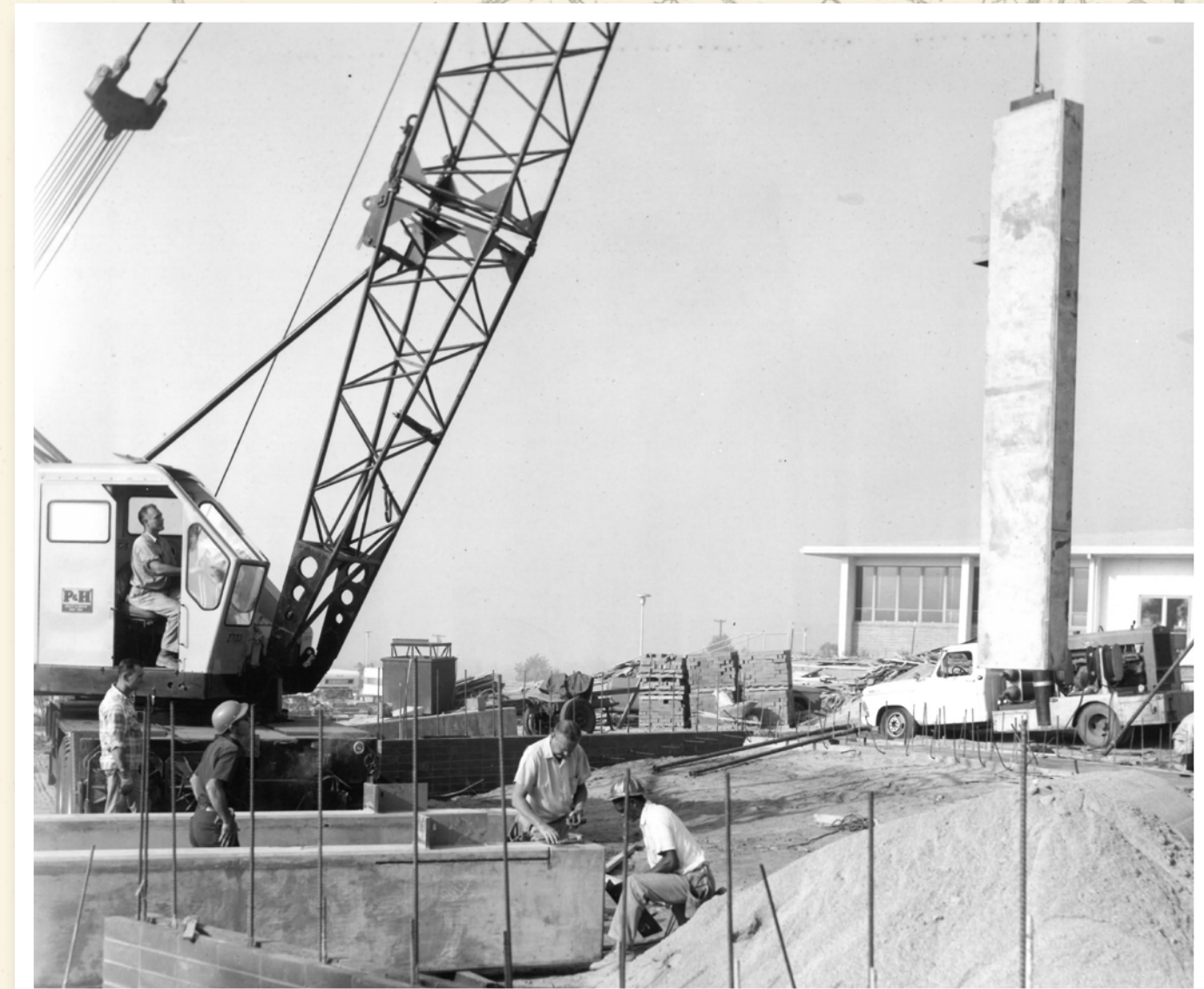
Wargin Hall under construction using tilt-up concrete piers.
